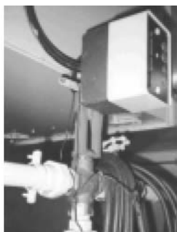
Thermostats control valve actuators or dampers
