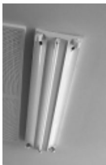
Triple tube fittings often only require one or two triphosphor lamps
