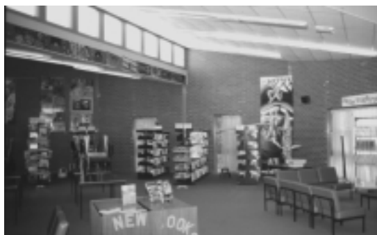
High windows reduce the number of lights used during daytime
